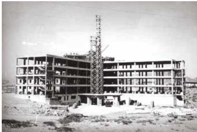
Construction of Providence in 1950 showing the core area and the wings. (Photo courtesy El Paso County Historical Society)
