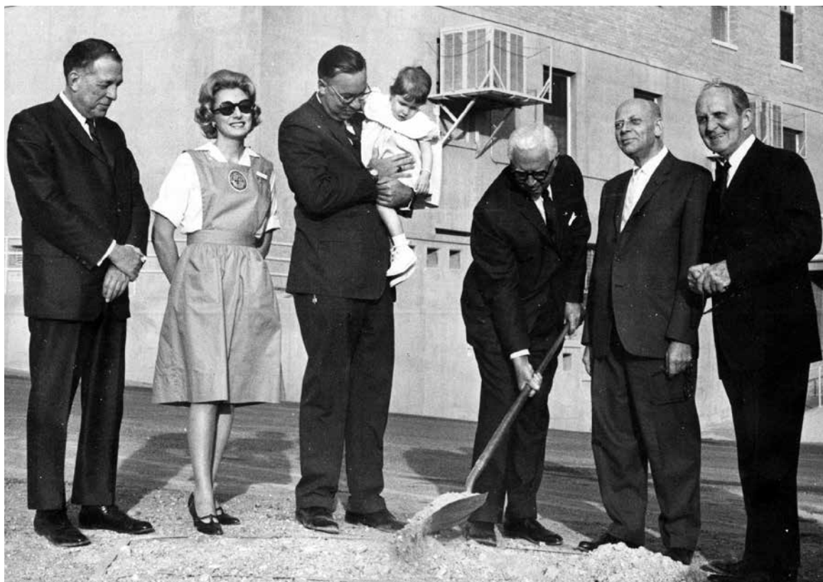
Sam D. Young, chairman of the Board of Trustees of Providence Memorial Hospital, turned the first shovel of earth for construction of the West Tower of the hospital. Taking turns at the shovel were from left, Dr. J. Edward Stern, president of the Providence medical and dental staff; Mavis Escobar, president of the Women's Auxiliary; Administrator Bob Byrne, who is holding Shelley Kidd, a lifelong patient; Young; Gus Bianche, executive vice president of Providence, and Dr. Paul Poling, hospital chaplain and director of public relations. (Photo courtesy El Paso Times )
